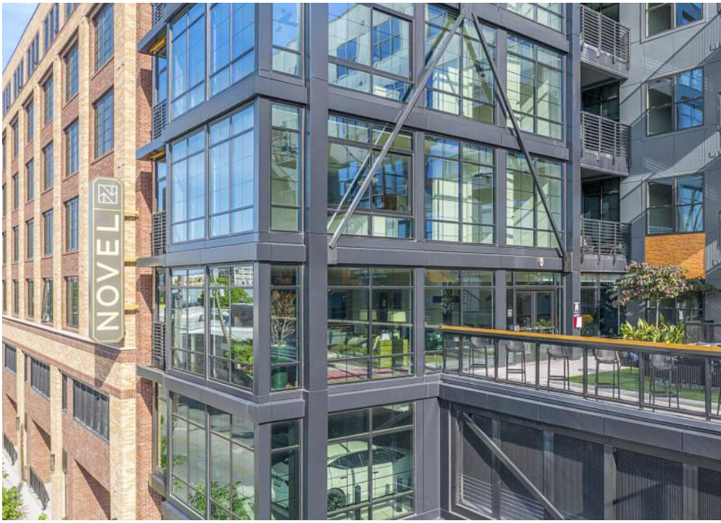
CROSS-BRACING: METAL PANEL + FIBER-CEMENT
